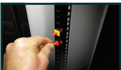
We wanted to ensure that mounting equipment up to 20kg (44lbs) was possible. With a safety factor of three, 60kgs (132lbs) was our target shear strength for one stud.
